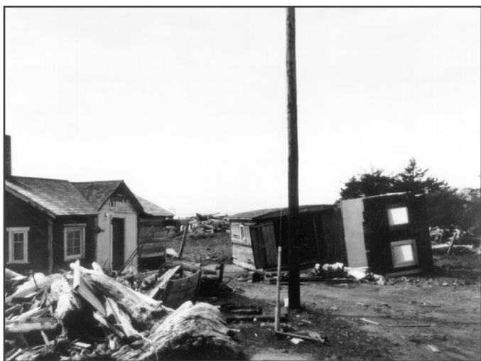
Figure 4. Damage to a medium-sized home in the town of Pacific Beach, Washington, from tsunami inundation during the 1964 Great Alaska Earthquake. The home was lifted from its foundation and a portion of the house was torn away. The entire house moved northwest 40 ft (12.2 m) from its foundation and parts of the yard were eroded and covered with debris. Photo from Hogan and others (1964).
