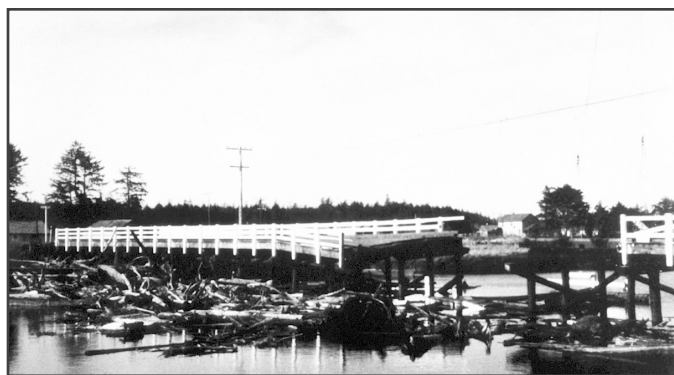
Figure 5. Destruction of the Highway 109 Copalis River Bridge, following tsunami inundation from the 1964 Great Alaska Earthquake. Two spans were lost, and timbers were bent. Two other 20-ft (6.1 m) spans are shown considerably deflected. Photo from Hogan and others (1964).
